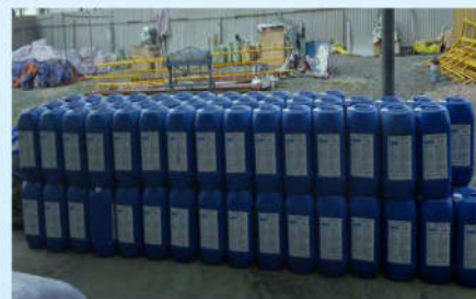
Xử lý ban đầu cho HVAC 6,000 RT Pre-treatment chemical at site HVAC 6,000 RT
